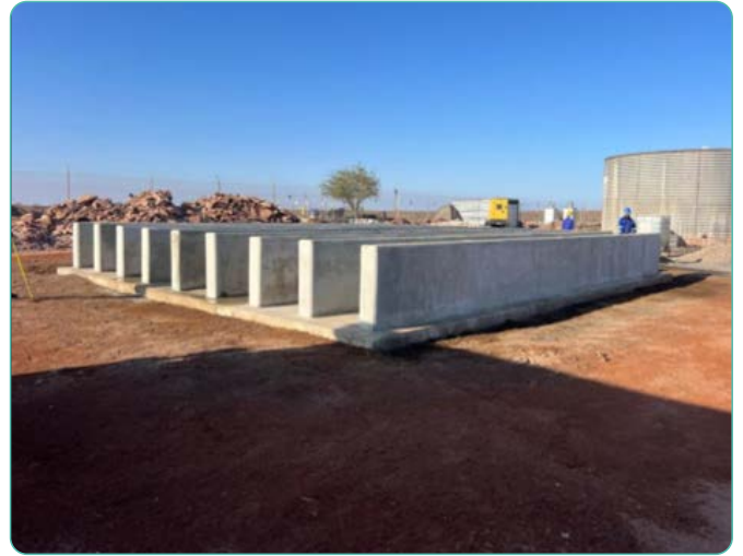
Photo: Foundation works for the new concrete reservoir, Aroab Extension and Upgrade project
