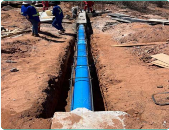
Photo: Encasement of pipeline, Aroab Extension and Upgrade project
