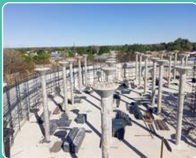
Photo: Ongoing work at Nkarapamwe 16ML Concrete Reservoir site.
